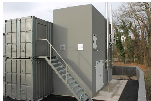
Doppelstock-Heizcontainer 2 x 90 kW Pellets, Industrie
